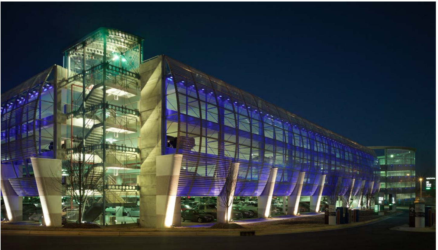
Charlotte Douglas International Airport— West Parking Deck
